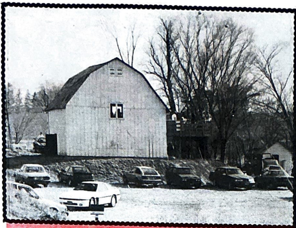
The Des Moines Rugby Football clubhouse is located in an undeveloped area south of Ashworth Road on 39th Street, West Des Moines.
