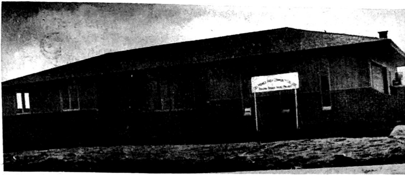
BUILDING Trades students recently completed this house at 801 S. E. 10th in Ankeny. Open house will be April 4, from 1 p.m. to 5 p.m.
