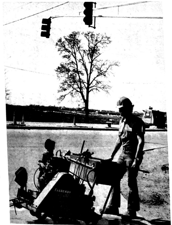
TRAFFIC lights recently went into operation at Oralabor Road and Ankeny Blvd. Jim Dickinson, of Oskaloosa, finishes up the construction.
