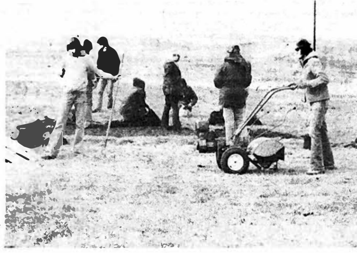
COMMERCIAL Horticulture students contribute much of their time and efforts in campus landscaping. They plant sod, trees and flowers. They grow and take care of plants in the Campus greenhouse. They also constructed the putting green east of Bldg. 25.
