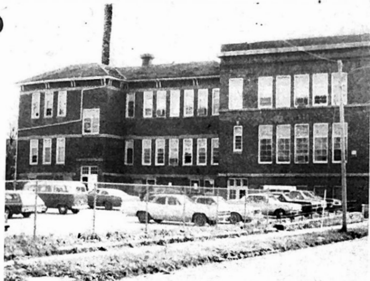
URBAN Campus students continue to seek improvements for their school. Administrators are working on a plan to move Urban Campus students into a Des Moines high school that is empty due to declining enrollment.
