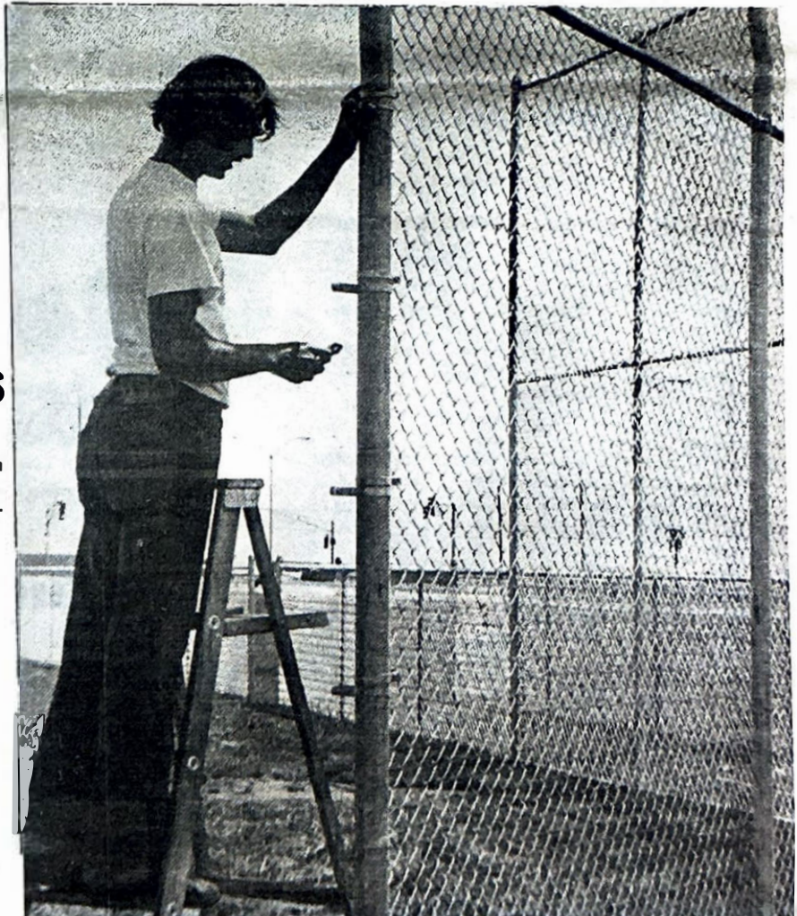
DON Moede finishes work on the fencing for the newly completed baseball diamond east of Bldg. 4.
